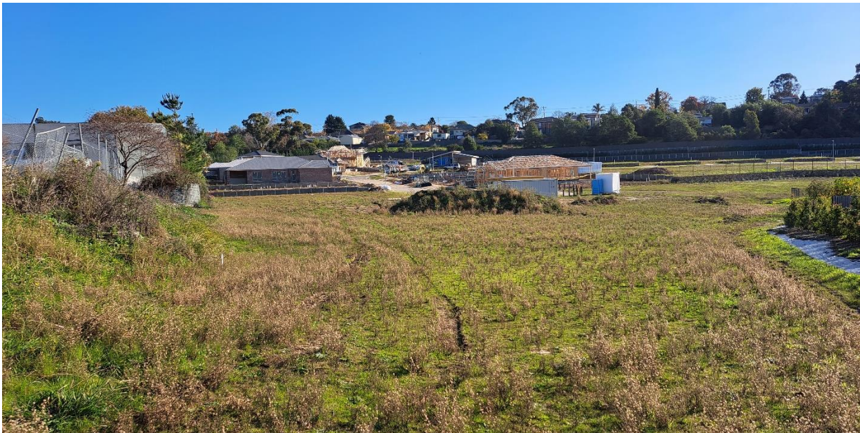
View of the 9 Janson site from higher east rear boundary towards the Janson court bowl. The site is free of vegetation where the proposed dwellings are to be constructed.
